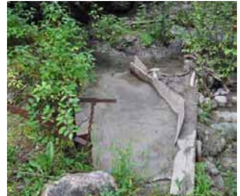
Boulder Creek Diversion Point
